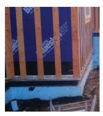
The exterior sheathing of the home was wrapped with a self-adhering vapor-permeable house wrap that serves as a weather-resistant air and water barrier. Furring strips were installed over this barrier allowing it to serve as a drainage plane for any bulk water that manages to get past the fiber cement siding.
